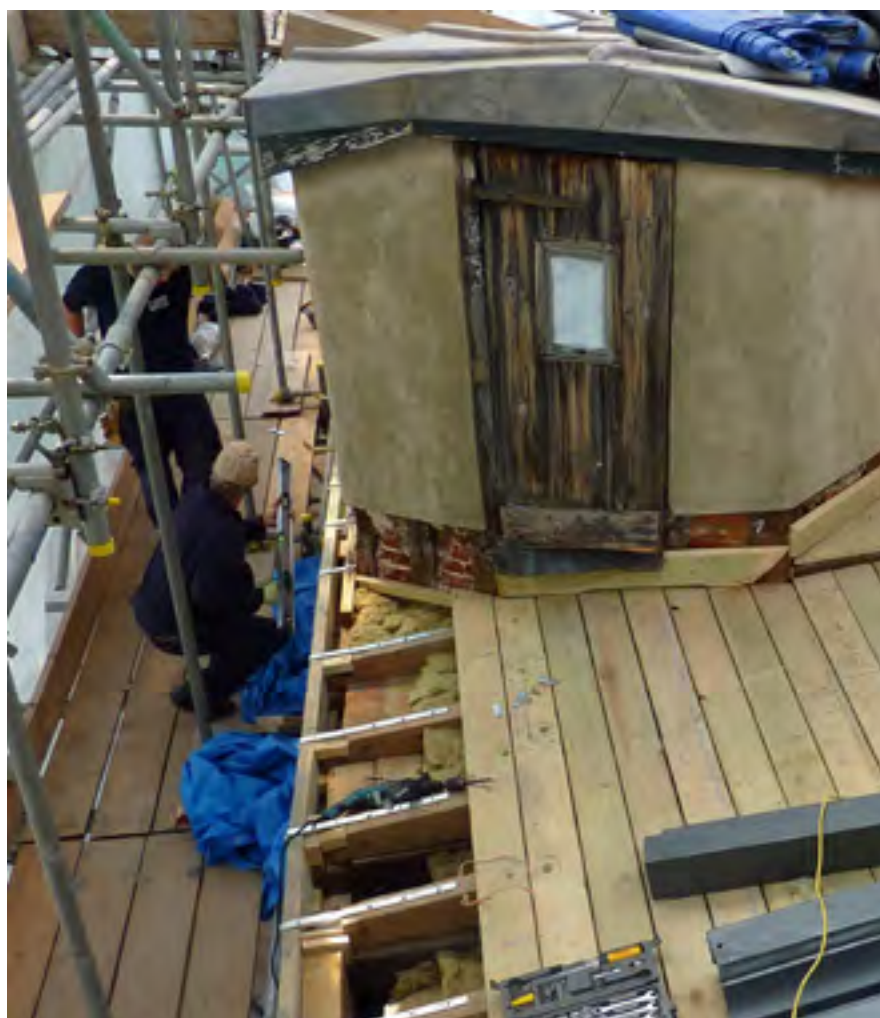
Technical drawing of a bat hotel at the Canons' Cloister, St George's Chapel, Windsor Castle and, below, construction in progress before the roof decking was re-laid
